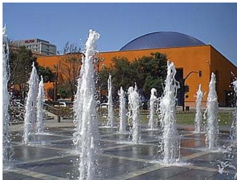
The 28,000 sq. ft. addition, complete with lecture hall, bistro and fountains sets the standard for the modern library
